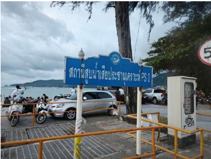
Figure 55. A wastewater facility near Patong Beach
